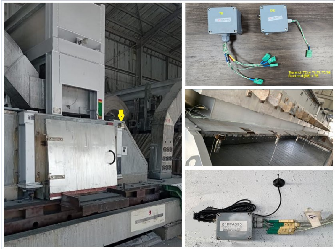
Figure 2. Installation of thermocouples and wireless sensors for cell preheat.
