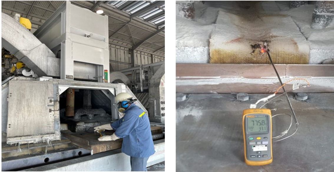
Figure 1. Manual temperature measurement during the cell preheating.
